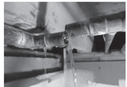
Picture of water pipes inside the wall. Water was leaking from a T-joint in the ceiling.
